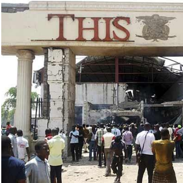
Plate 2: Thisday office bomb Blast, Abuja
