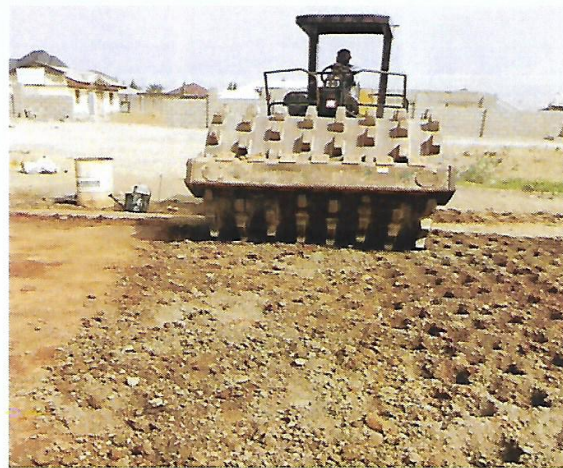
Figure 4: Compaction of the test sections using sheep-foot roller
