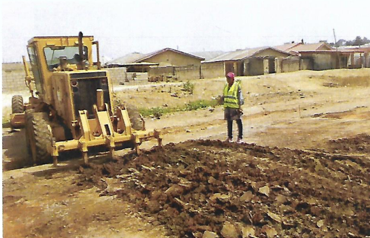
Figure 2: Scarification of the test sections using ripper
