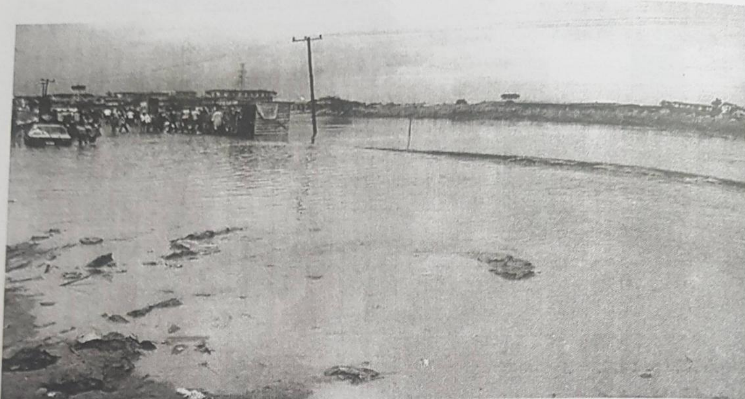
Plate 1: Properties and access road submerged by flood
