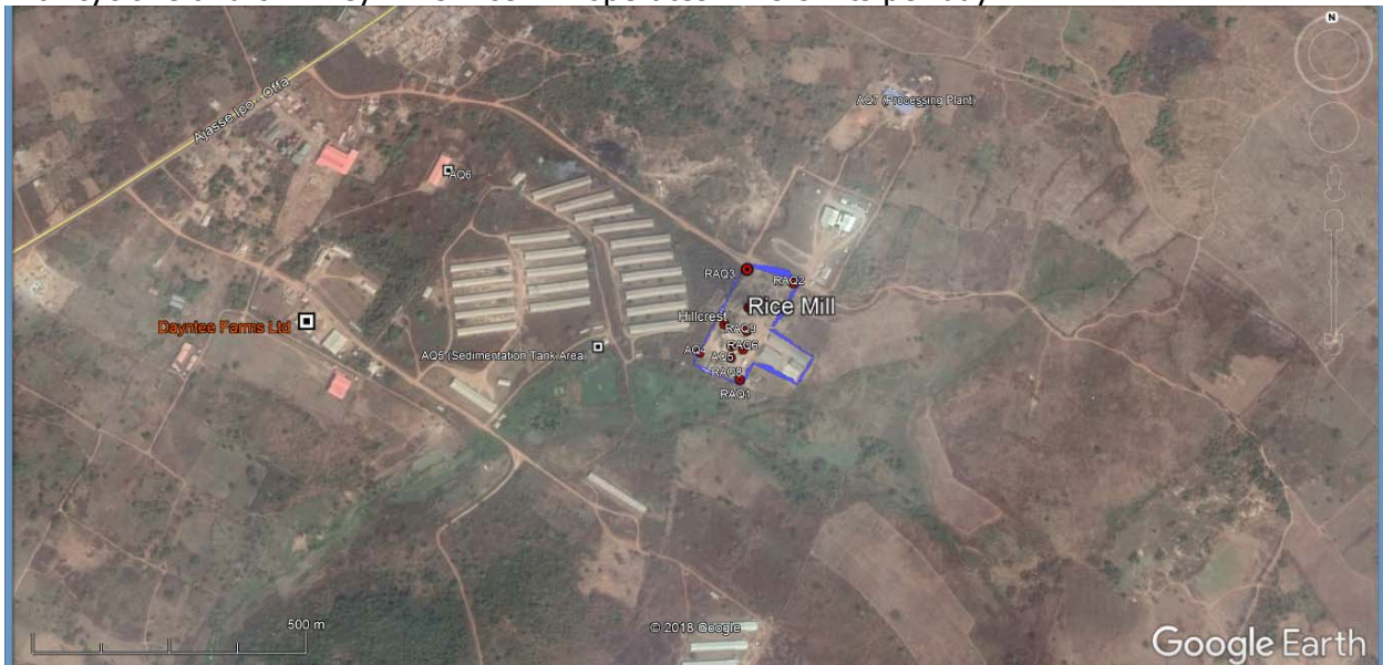
Figure 1: The Rice Mill Facility Site and Area of Influence
