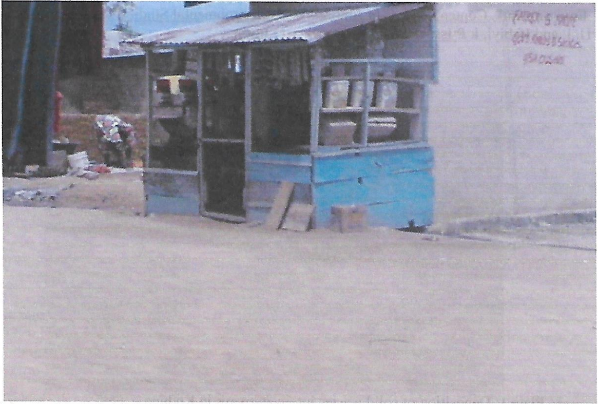
Plate 3: Construction of illegal structures on drainage channel at Sabon Gari, Zaria.
