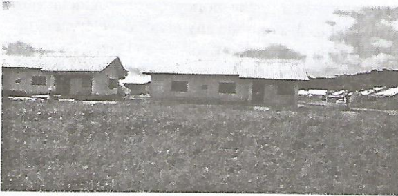
Plate III View of Dei-Dei resettlement housing scheme Source: Author's field work, 2011
