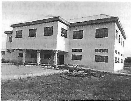
Plate III: Use of windows and low application of vegetation at FUBK Birnin-Kebbi
