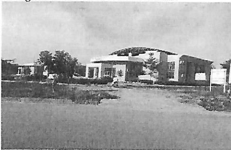
Plate V: Faculty building with vertical shading horizontal shading device
