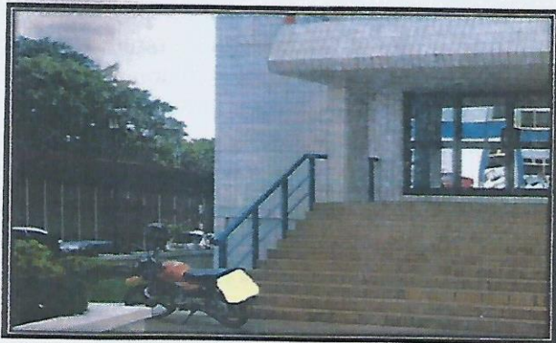
Figure 1: Entrance of a public building with no ramp provided Source: Authors Field Survey, 2014.
