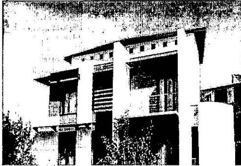
Plate 1: Approach facade of the Blasco House Source: Behance.net (2012)
