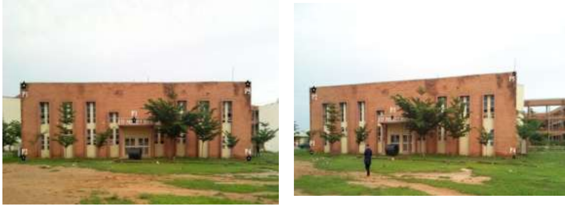
Plate 3: Images from Tecno W3 camera Left and right position capture, with structural control points identified
