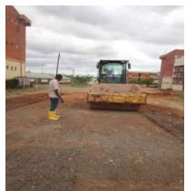
Fig. 8: Field compaction in progress
