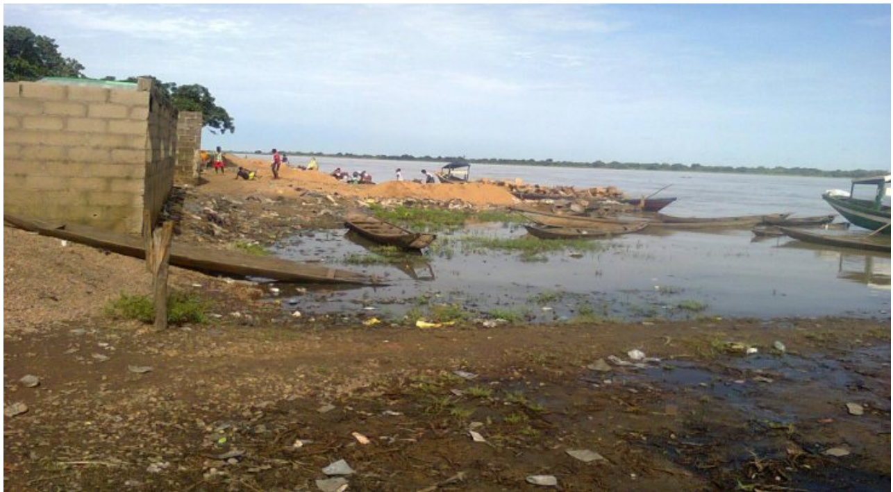
Fig. IV: shows an ongoing construction on the bank of River Benue (source fieldwork)
