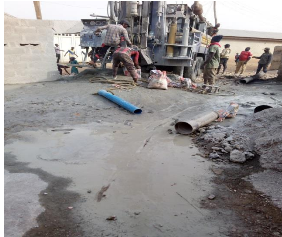
Plate IV. Granite Chippings for gravel packing. Plate V. Inappropriate Gravel packing of a borehole
