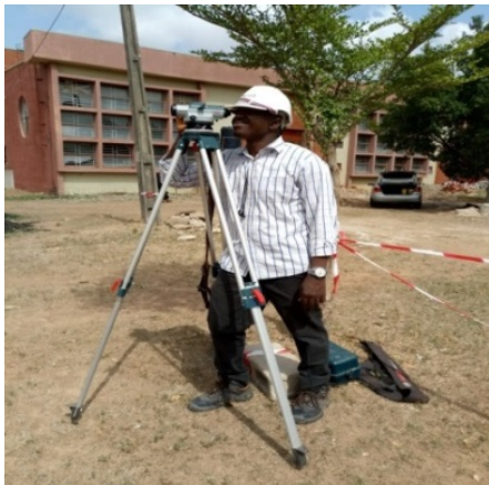
Fig. 6: Theodolite for leveling of subgrade
