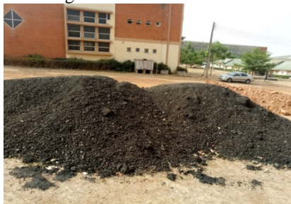
Fig. 2: Pile of milled RAP
