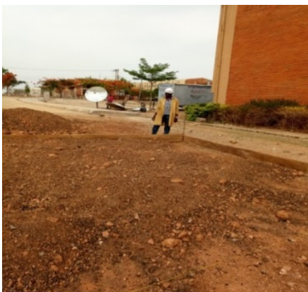
Fig. 7: Sections demarcated with planks
