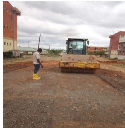
Fig. 8: Field compaction in progress
