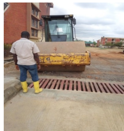
Fig. 9: Boundary with the existing pavement
