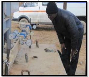
Fig.4: Taking Settlement Reading on Dial gauges
