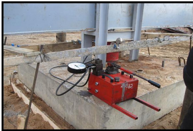
Fig. 3: Loading device for field investigations (200Tonnes capacity)
