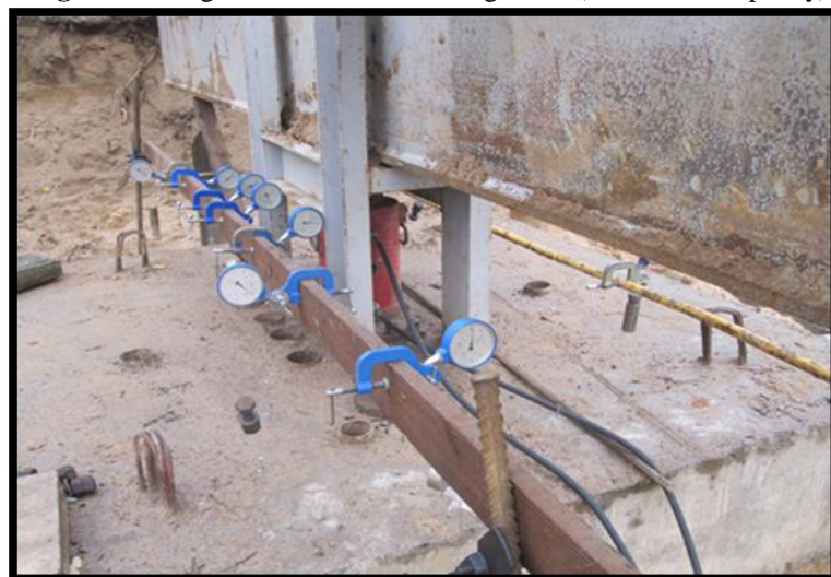
Fig. 4: Dial gauges for sensor movement measurement under pile cap
