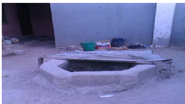
Plate 2. An open hand-dug well in Zango Local Government Area of Katsina State, Nigeria
