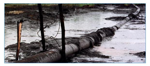
Plate 1: Land degradation due to leakage from crude oil pipeline in the area
