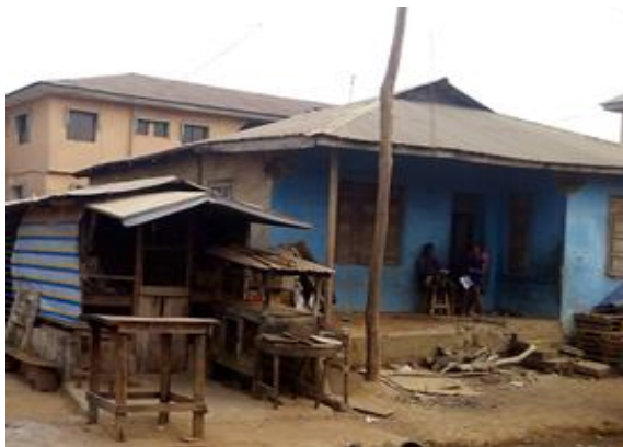
Plate 4: Kitchen/toilet positioned beside a rear side of the building
