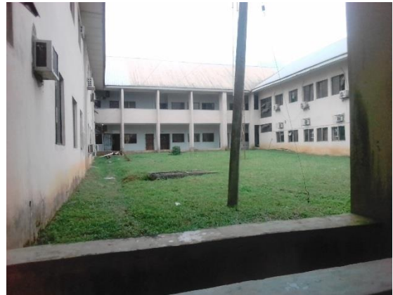
Plate vi: View of the courtyard Source: Author's field work (2017)
