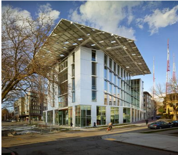
Plate 7 – The Bullitt Center, Seattle, Washington, USA Source: https://www.archdaily.com
