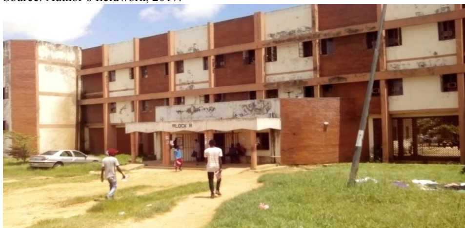
Plate 1 Hostel Building with littered environment and not renovated Source: Author's fieldwork, 2017.
