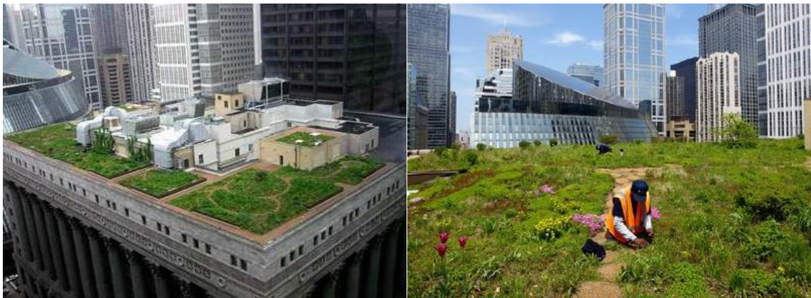
Figure 5: Chicago's City Hall Green Roof
