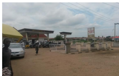
Plate II; First El-Shaddai Nig. Ltd shares boundary with another Filling Station and market For farming
