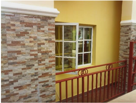
Plate IV: Casement window at Princess Ah-zahra lodge. Source: Author's fieldwork, 2017.
