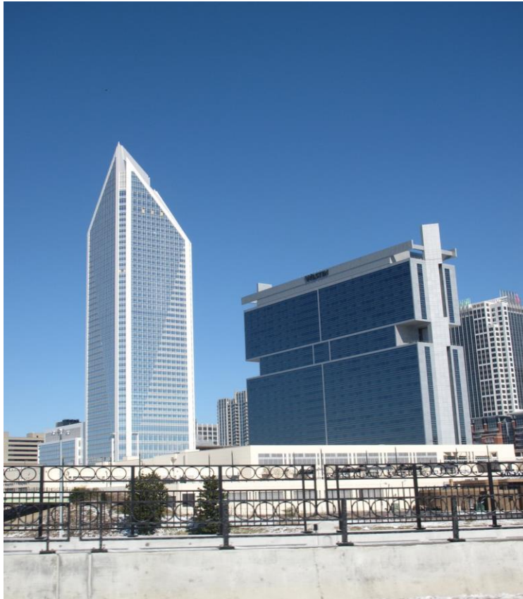
Plate 12: The Duke Energy Center, Charlotte, North Carolina, USA
