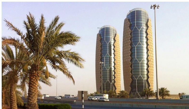
Plate 5(a): Al Bahr Towers, Abu Dhabi Source: 7 Intelligent Buildings (2017)
