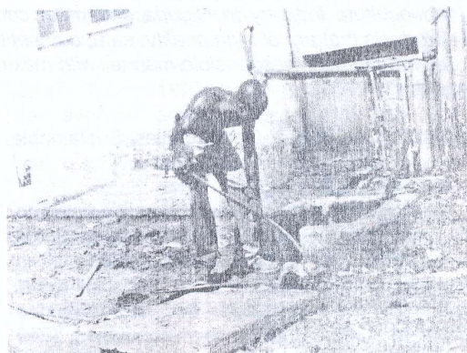
Fig 5 De-silting of manhole
