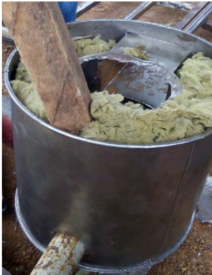
Plate I: The stove wall insulation process
