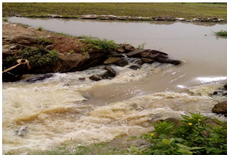
Figure 4: Distribution canal Failure in Kontagora scheme.
