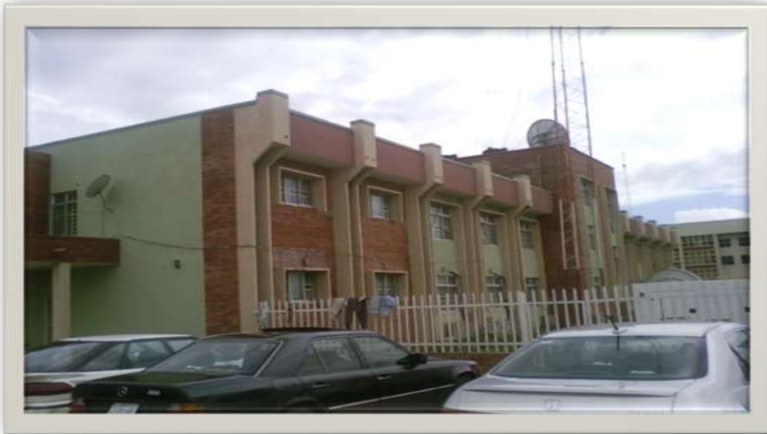
Plate V : Showing the Rear and Side View of the Building
