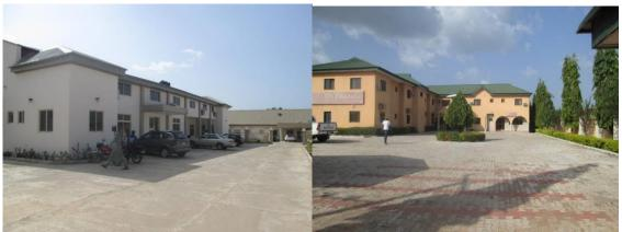
Images Showing a Stand-off less than 5 meters at Haske Luxury and Yayi Hotels Respectively.
