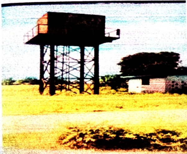
Plate 5: The Water Tank and Pump House
