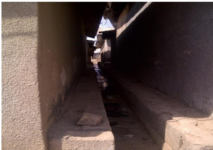
Figure-3. Houses Built on Drainage Network
