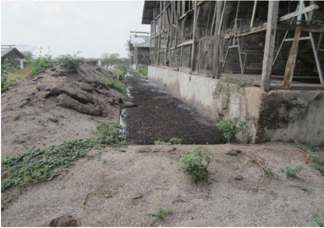
FIGURE 7 Open drain Poultry waste disposal method
