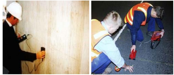
Figure 2- Cover meter measurements, concrete column (Left) and concrete deck overlaid with asphalt (Right)
