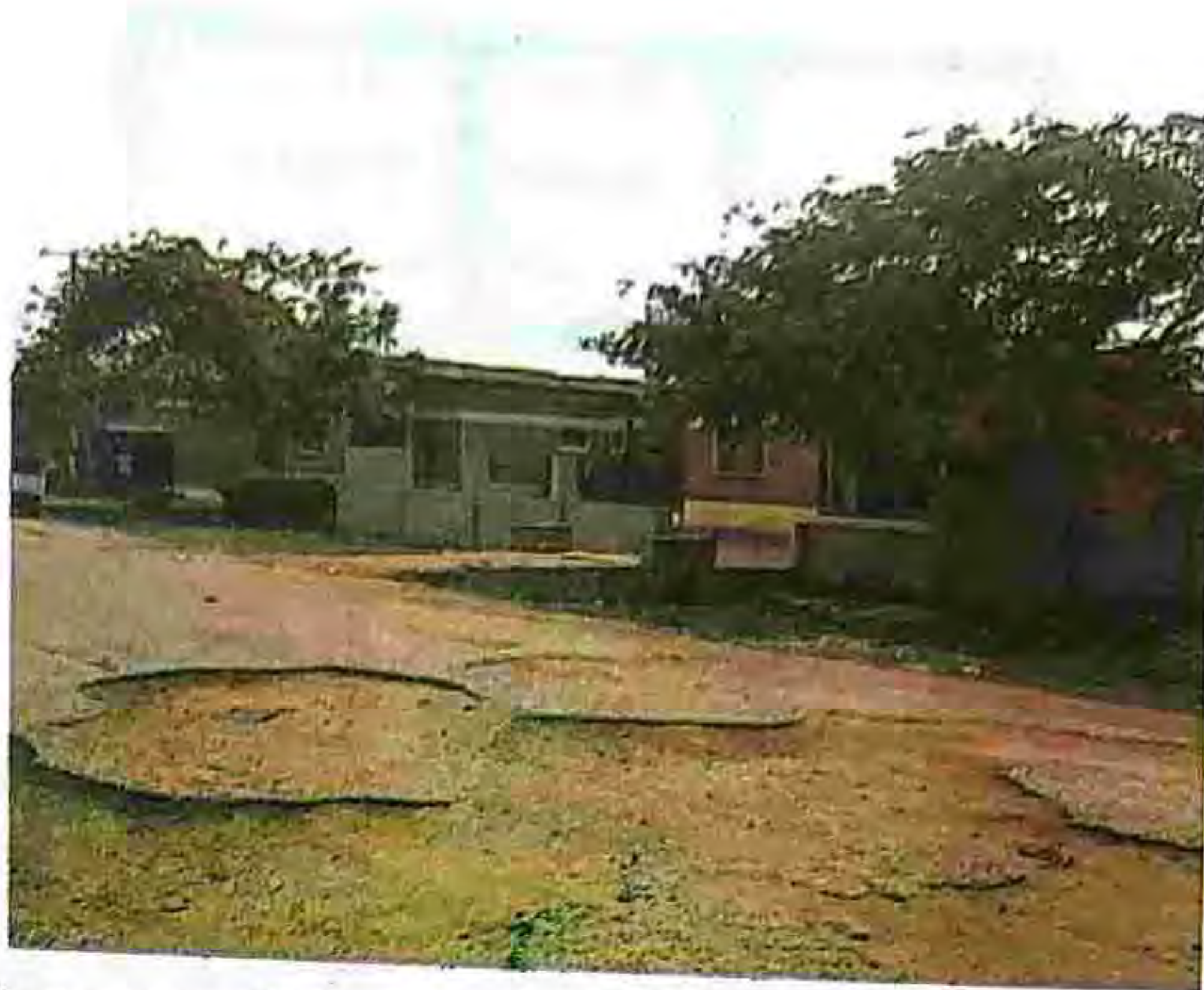
Plate 4: Showing a row of 3 bedrooms at Bosso Estate. Source author's survey 2011
