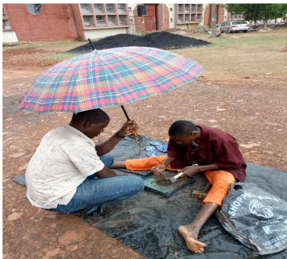
PLATE VI: IN-SITU DENSITY TEST OF RAP
