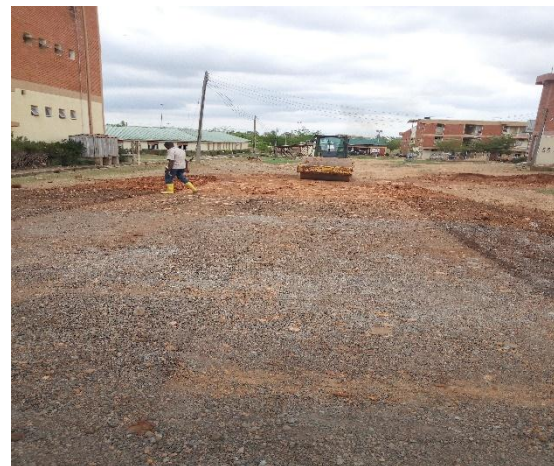
PLATE III: FIELD COMPACTION OF LATERITE-RAP MIX
