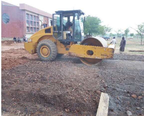
PLATE IV: FIELD COMPACTION OF LATERITE-RAP MIX
