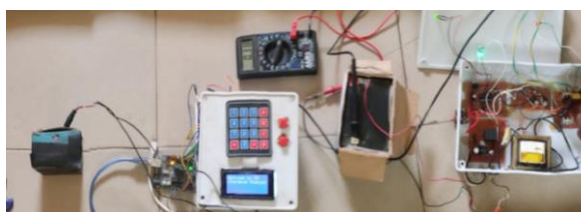
Figure. 8. The Metering System with the Electric Vehicle Charging Hub
