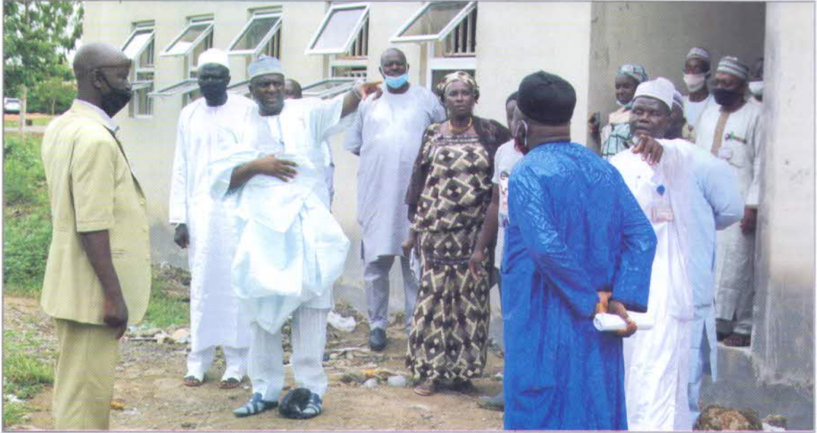
The VC, Prof. Bala (m) explaining a point to the contractor at the site while others watched with keen interest.
