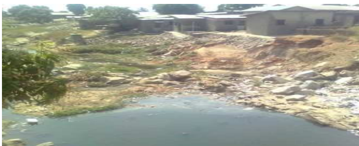
Plate v: Showing an erosion site along Mypa Bridge
