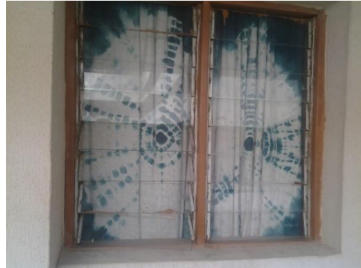
Plate 4: louvers window Source: Author's fieldwork (2016)
