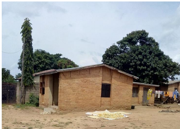
Plate 1.0: Housing units at LMAH.
