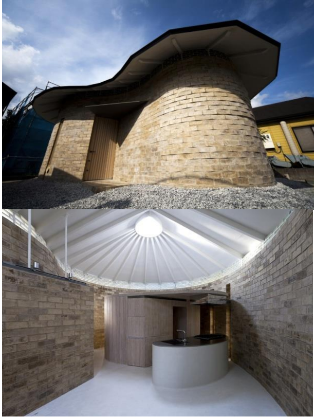
Plates XXIV & XXV : Exterior and Interior views of the Earth Brick Residence in Chiba, Japan. Compressed Earth Bricks applied on walling Source: Rael (2009). Earth Architecture
