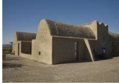
Plate XV: Rammed- earth Housing, isle D'Ábeau, France. Applied on the floor, wall and roof.
