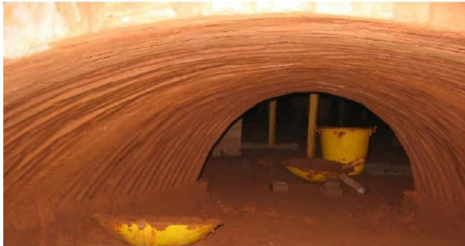
Plate XXIII: Vault (with compressed earth blocks) connecting between a segmental arch and a semicircular arch. Source: Rabie (nd). Auroville Earth Institute
