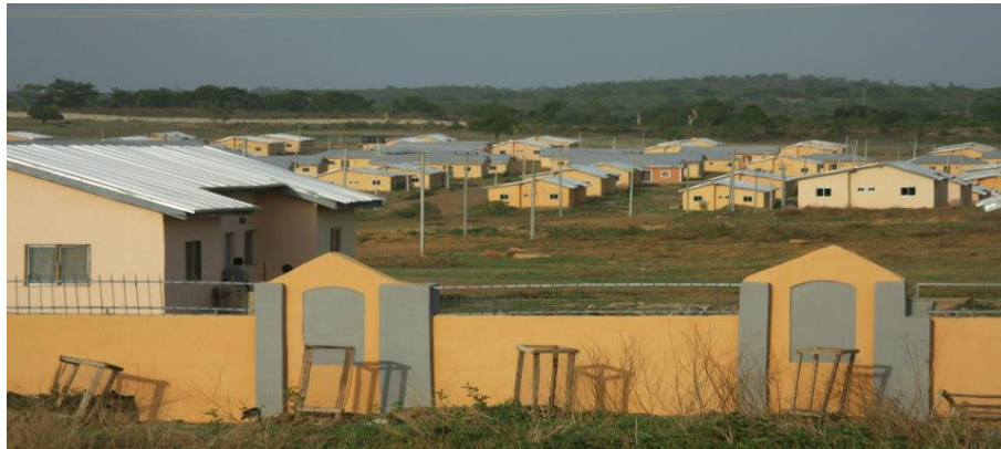
Plate 2: The site after construction
