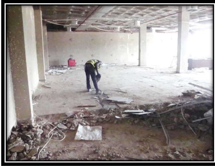
Plate 1: Removal of Floor Finish using powered tools Source: Author field Survey (2015)
