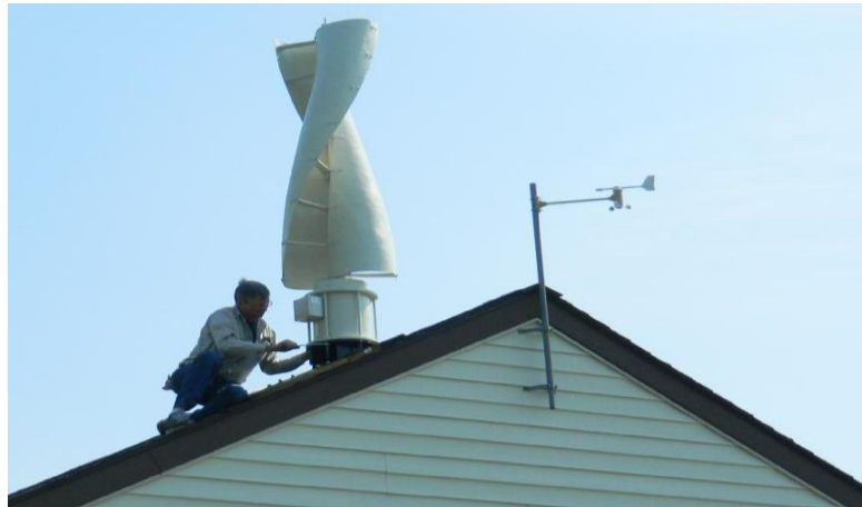
Portable Vertical Axis Wind Turbine (Mounted on a Roof)
