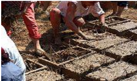
Plate VI: Mixing mud and straw in brick frames Source: Wikipedia (2015).
