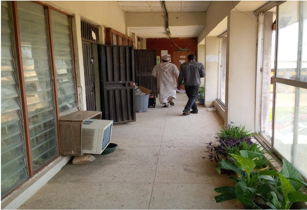
Plate iii showing balcony in a faculty building of State Polytechnic Zungeru
