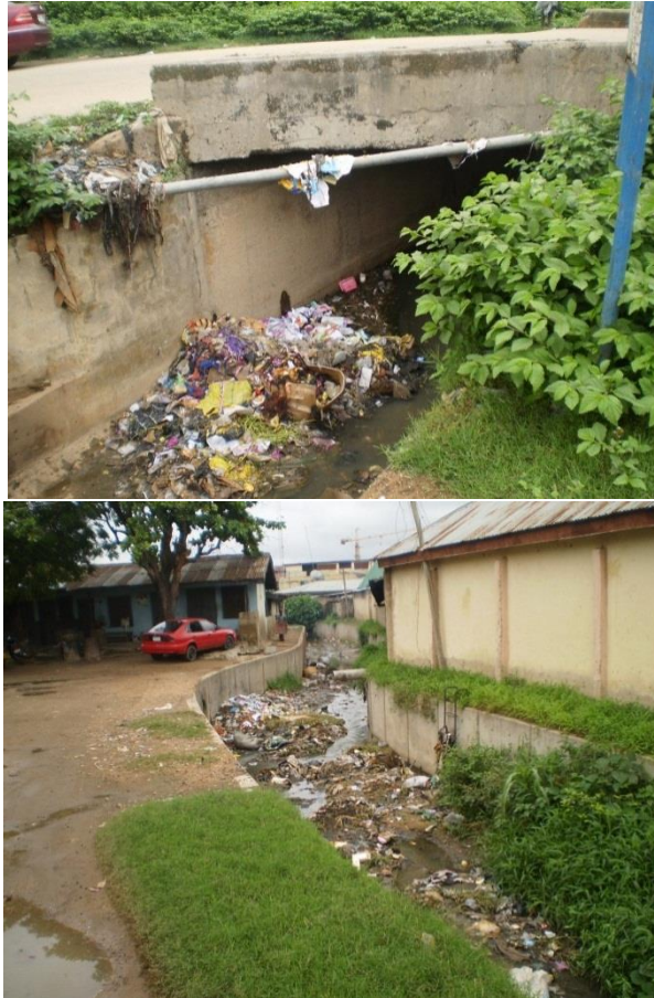
Plate 2 and 3: A drainage line with deposits of solid wastes. Source: Researchers field work (2015).
