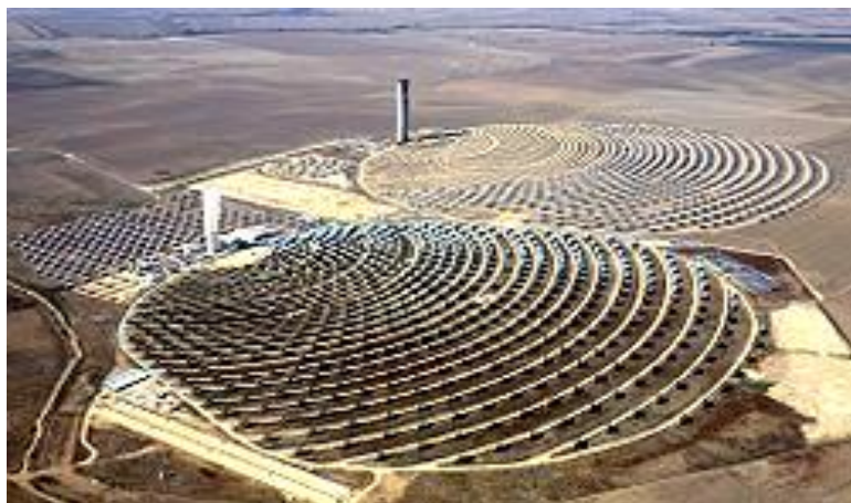
A Typical 100mw Solar-Power-Plant on 650acres of Land (Enough to Supply 30,000 Homes)
