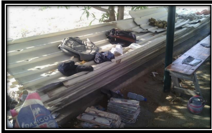
Plate 3: Roofing sheets carefully salvaged. Source: Authors Field Survey (2015)
