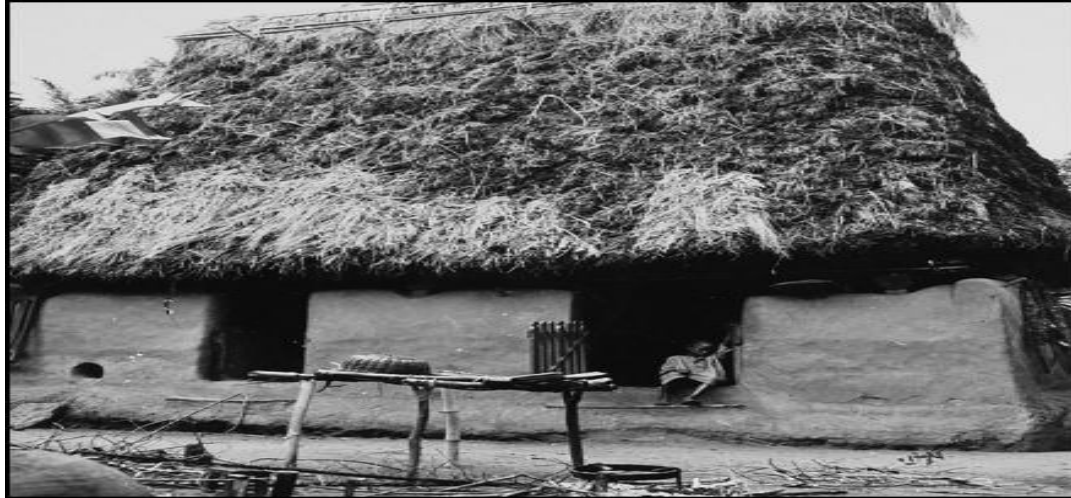
Plate I: Traditional Building in Anambra State, Showing Thatch-roof on Load-bearing wall system. Source: Tropenmuseum (1967).
