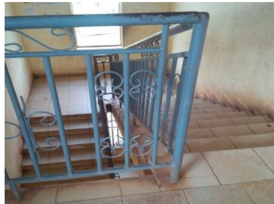
Plate 7: Emergency Stairway of Male Hostel Badamasi Babangida University Source: Field Work (2015)
