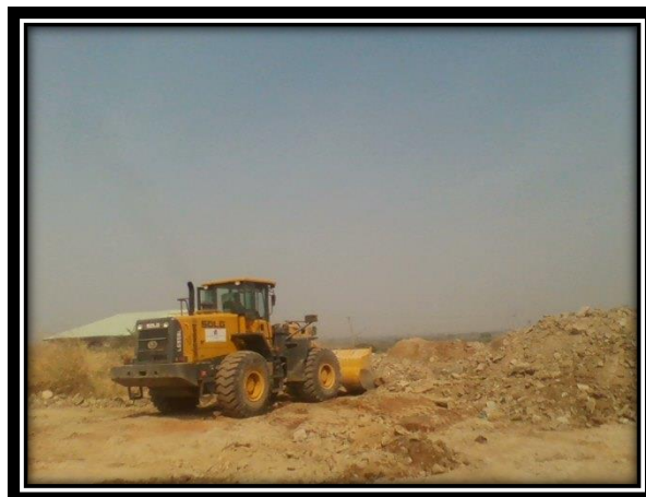
Plate 4: 'Bulldozer approach' used in demolishing structural waste. Source: Authors Field Survey (2016)
