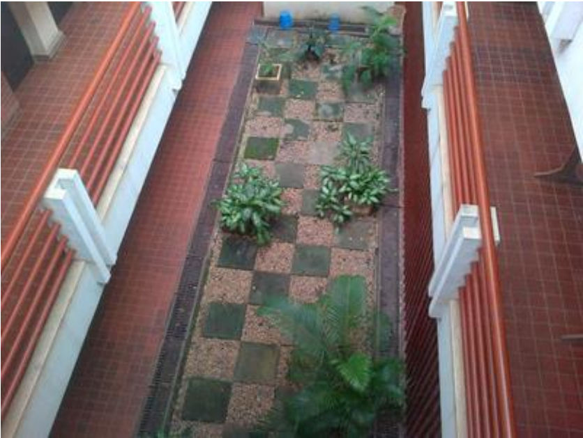
PLATE 3: showing the courtyard. Source: researcher field work (2015).
