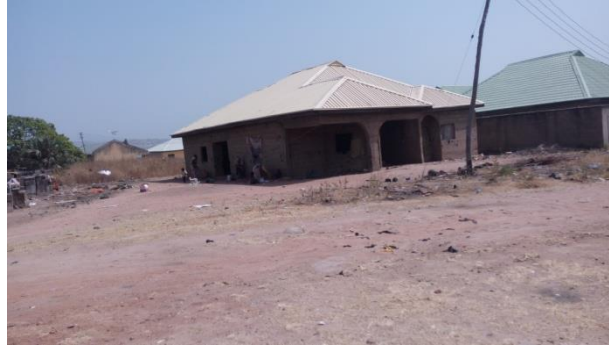
Fig3.0: An abandoned building in London street 1 occupied by illegal occupants
