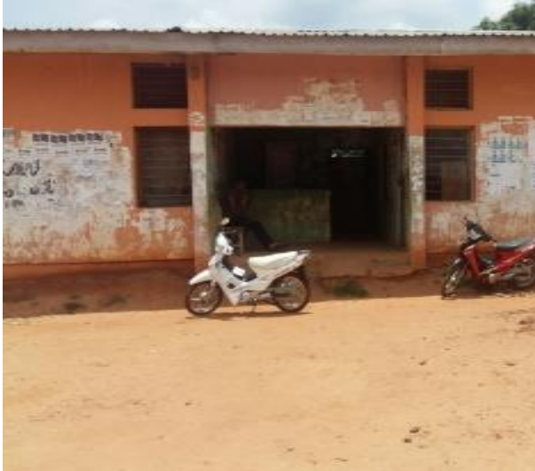
Plate 8: Entrance of Male Hostel Federal Polytechnic Source: Field Work (2015)
