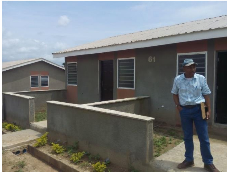
Plate 2: Housing units at FFAH.
