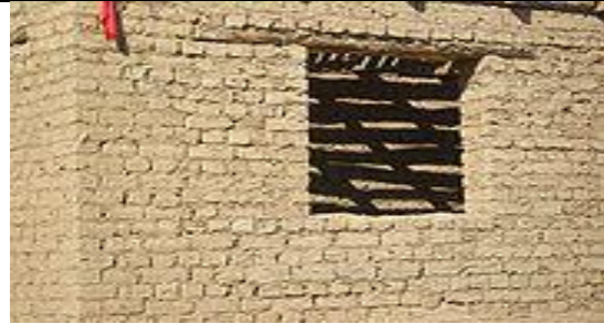
Plate VII: Adobe brick house under construction
