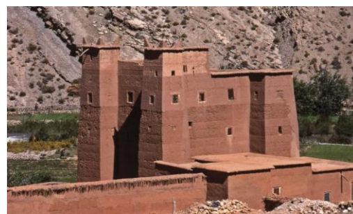
Plate XIII: Five-story Rammed-earth Building in Morocco; walling and roofing.
