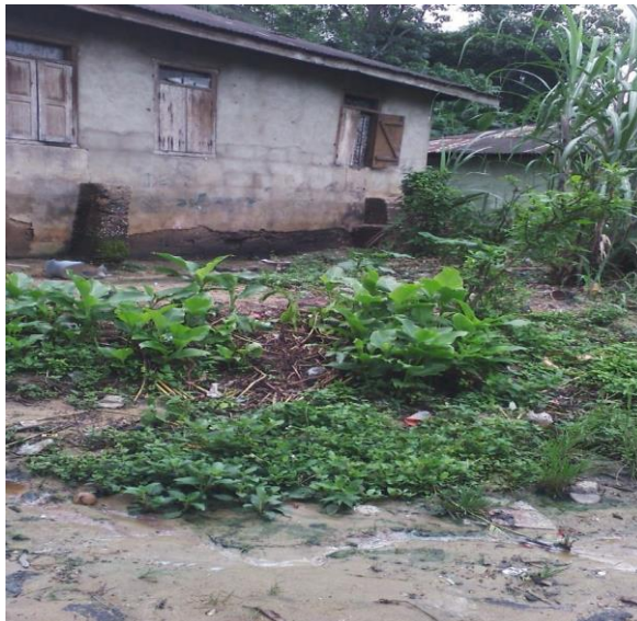
Pillars made of Concrete mix of Shells, sand and cement to Support Already Washed and Exposed Foundation of a
