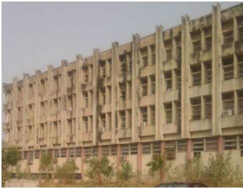
Plate 1: exterior view showing vertical Fins
