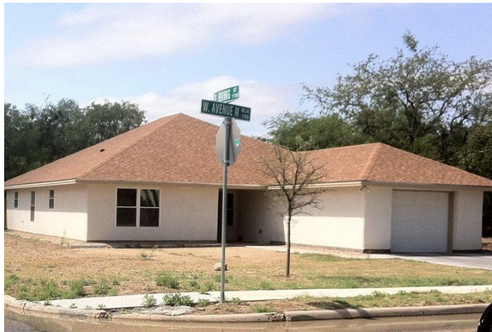
Bungalow Constructed With Compressed Earth Bricks
