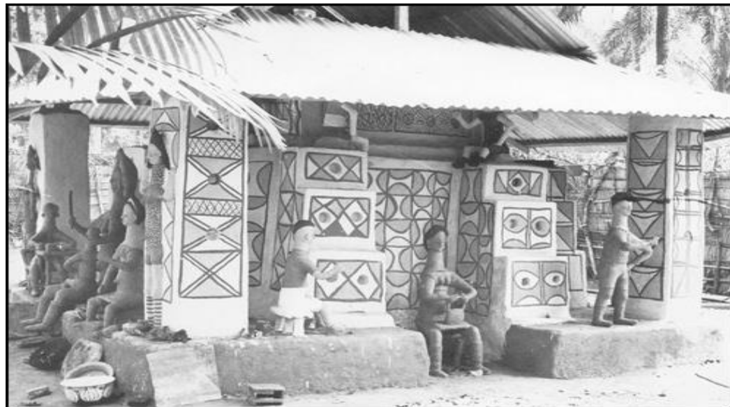
Plate I: Traditional Building in Anambra State, Showing Thatch-roof on Load-bearing wall system. Source: Tropenmuseum (1967).
