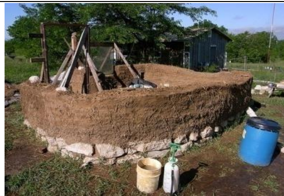
Plate II: Cob construction process.
