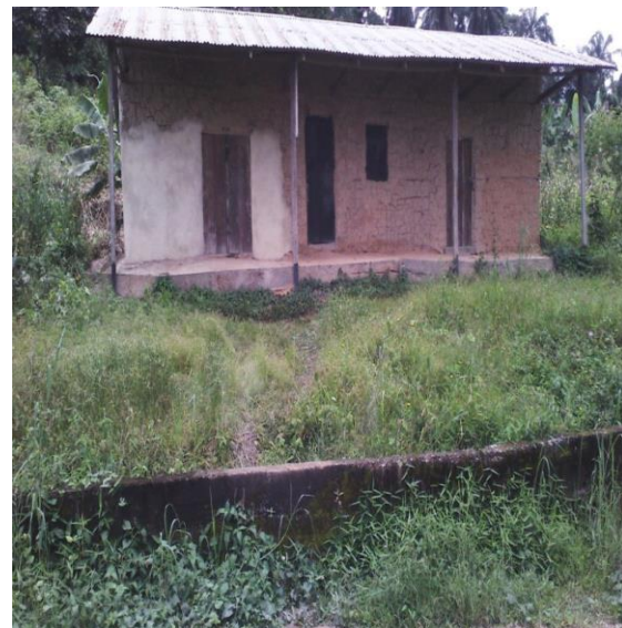
Barrier and Contour Constructed in Afia Isong Community to Restrict Flood Water
