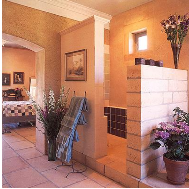
Interior of a Bungalow Constructed with Compressed Earth Bricks
