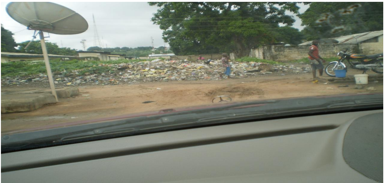
Plate 9: An open dump servicing Police Barracks Source: Researchers field work (2015).
