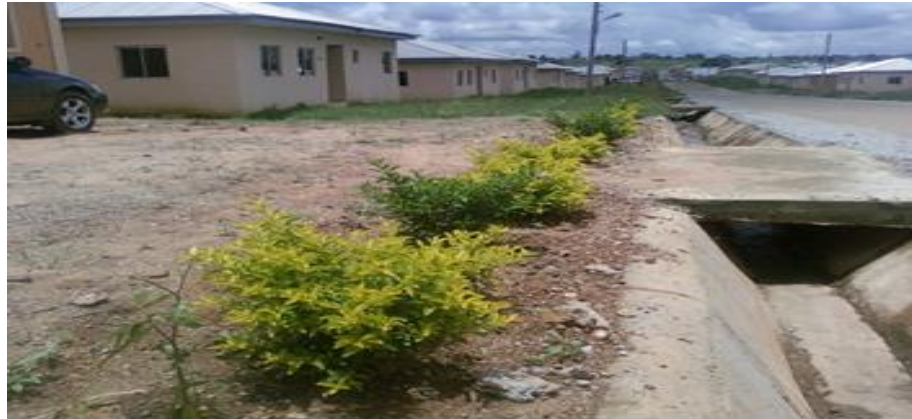
Plate 3: The site after construction, showing the road, drainage and planted shrubs
