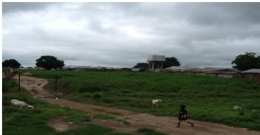
Overhead Water Tank and Telecommunication Mask
