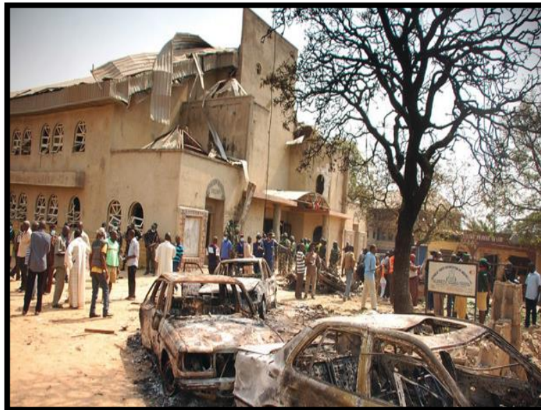
Plate 1: The bomb effect on the building of St Theresa church at Madalla
