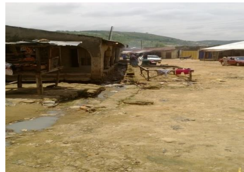
Plate II: Open gutter in Maitumbi, Minna. Source: Author, 2014
