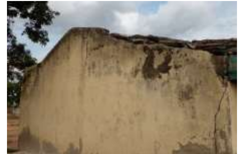
Plate 12: Showing dilapidated eaves and parapet
