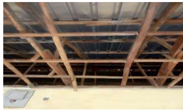
Plate 2: Showing corridor without ceiling
