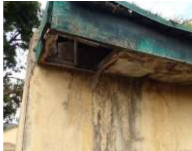
Plate 12: Showing dilapidated eaves and parapet
