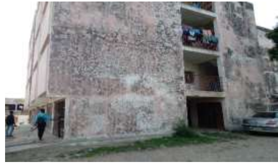
Plate 13: Showing faded walls and collapse fence
