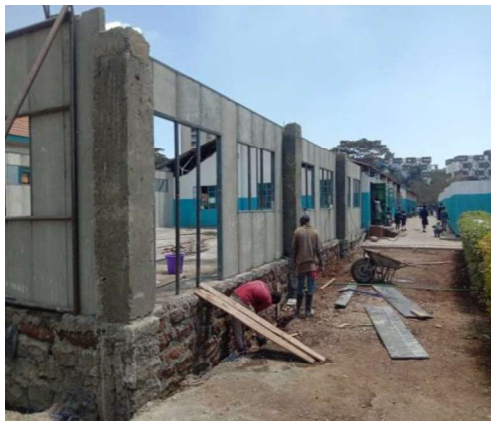
Figure 11: Precast Concrete Wall wall
