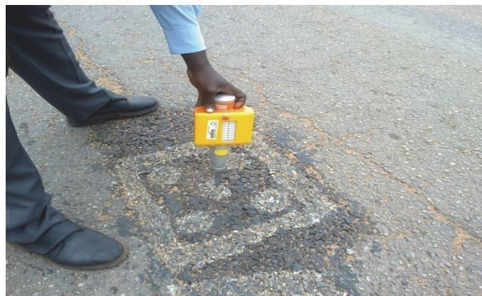
Figure 3: Rebound hammer test
