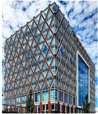
Plate II. The use of low solar gain low-E double glazing in Marble David building Source: Mueller (2005).
