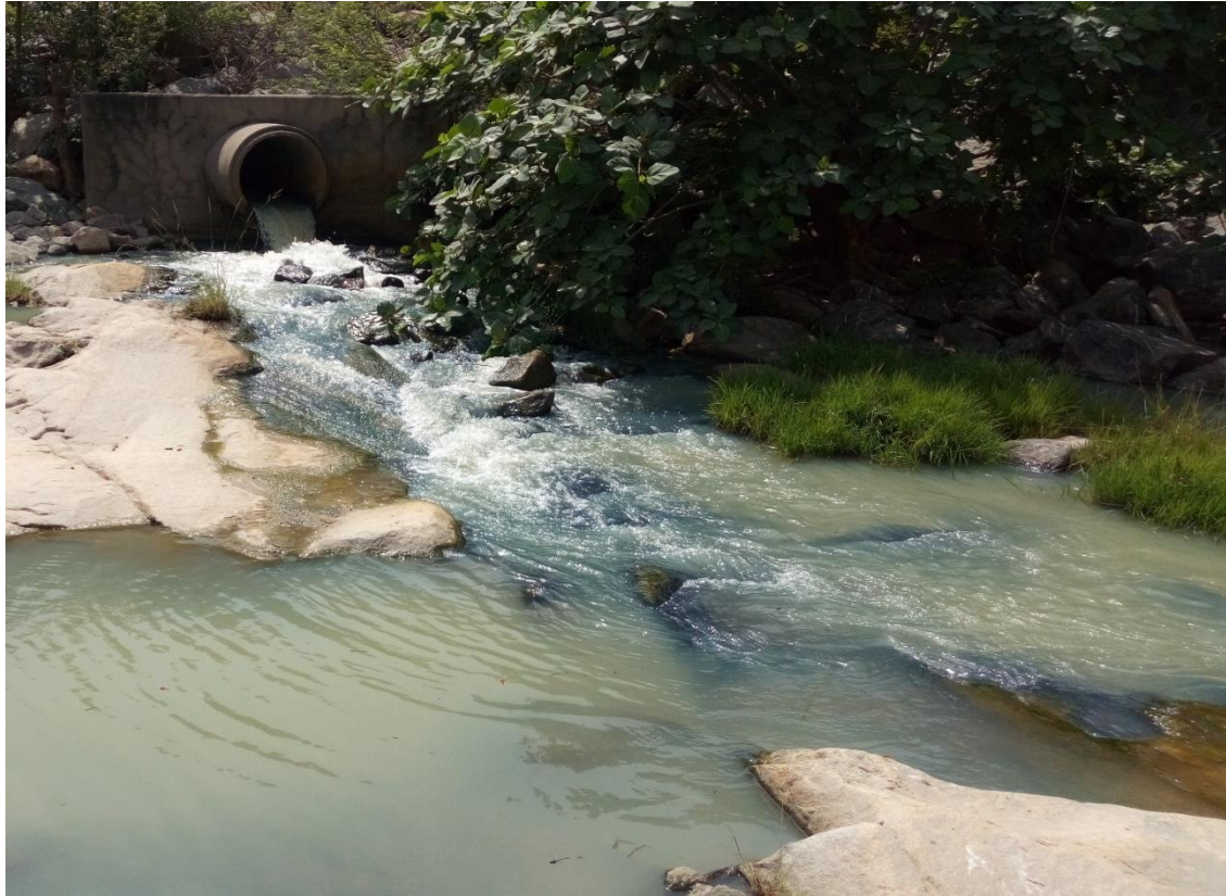
Plate IV: Drainpipe into River Kaduna at Shiroro Dam
