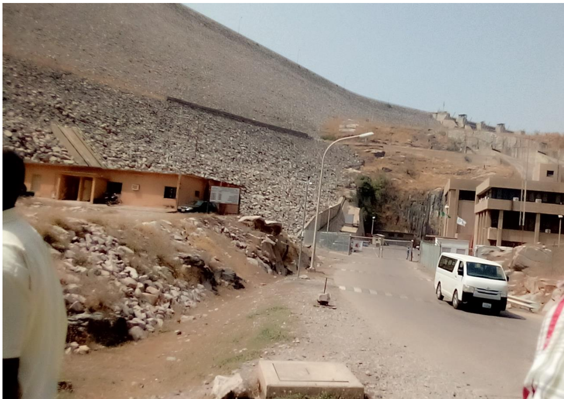
Plate III: Shiroro Hydropower Office Building
