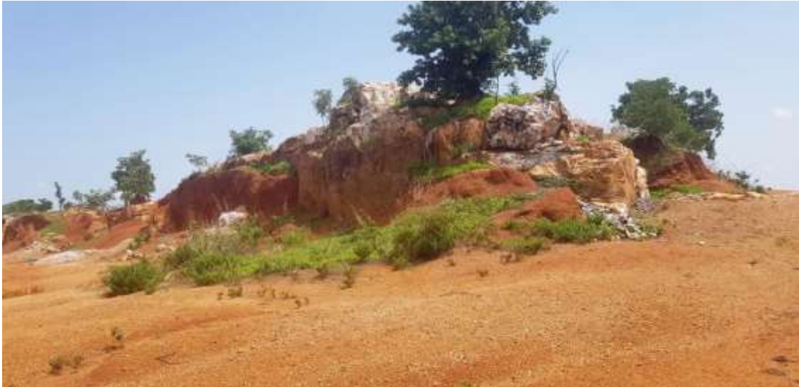
Plate V: Quartzite outcrop excavated for rock aggregates. Location coordinates (N 08° 40' 56.4", E 08° 32' 45.2", 223m ASL)
