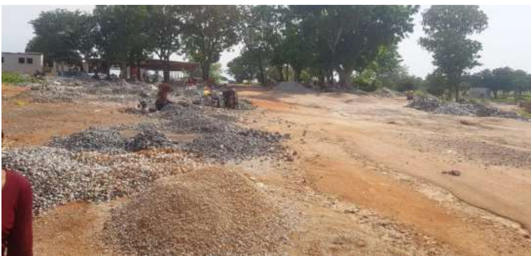
Plate XI: Women involved quarrying overburden rocks into rock aggregates
