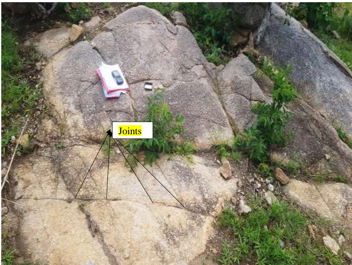
Plate XXII: Cross-cutting Joints on porphyritic granite at Lakwanti Yakoko (8°57'57.5"N, 11°41'36.9"E)
