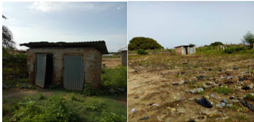
Figure 9. Public toilet at Garatu and Gidanmangoro rural communities, respectively
