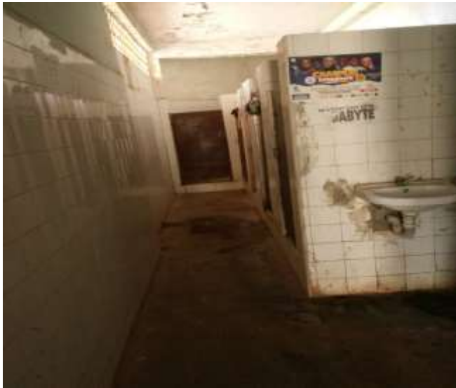
Figure 4.6 Block B Male Hostel Toilet
