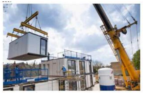
**Figure 2.1: Installation of Modular Home** Source: Wuni *et al.* (2019)
