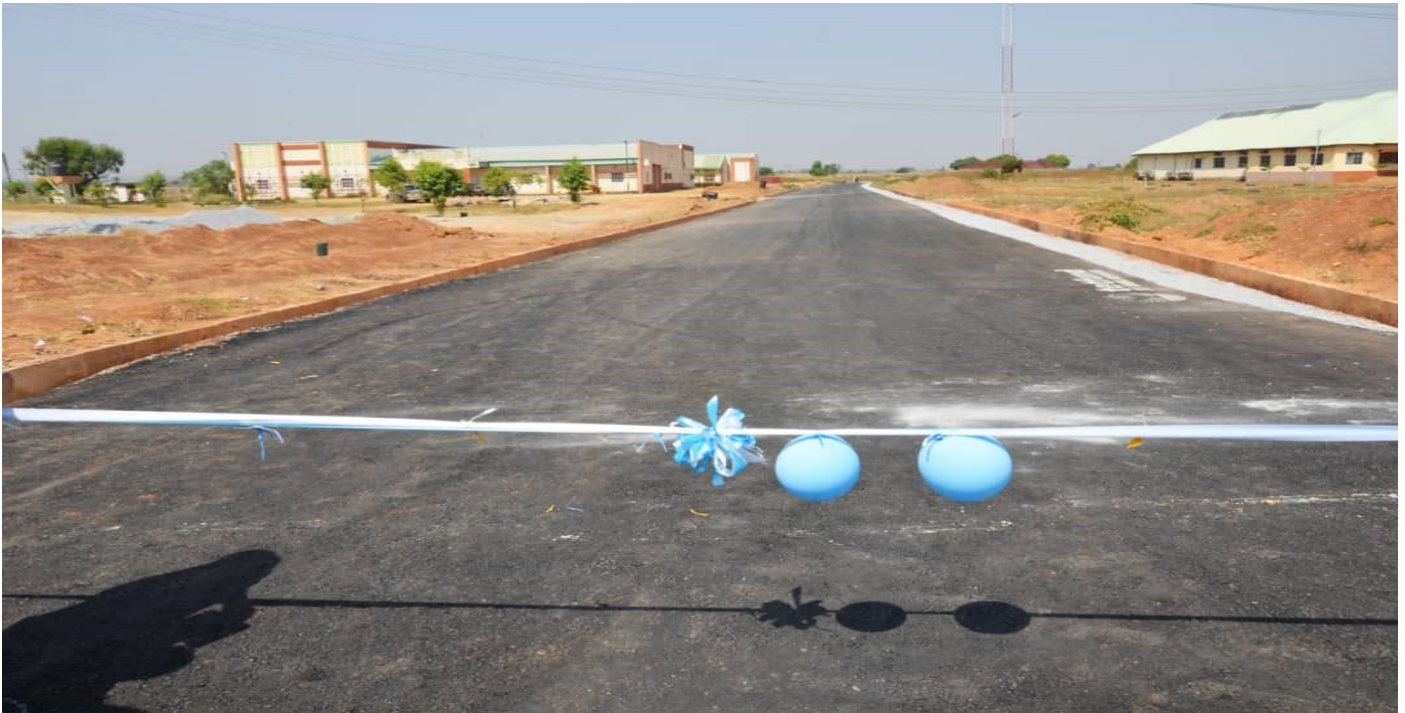
The newly constructed road.
