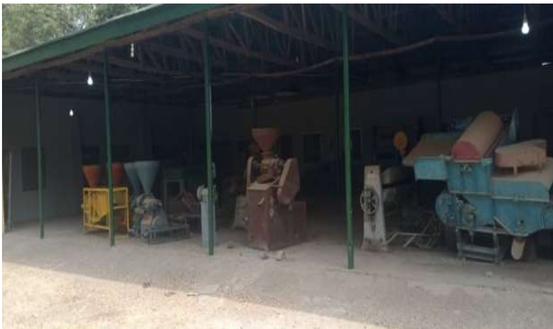
Plate V: Dilapidated Rice Processing Machines in the Study Area
