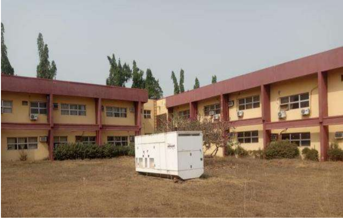
Plate III: A 27KVA Mikano Generator Set used to power the office complex of the National Cereals Research Institute (NCRI), Badeggi
