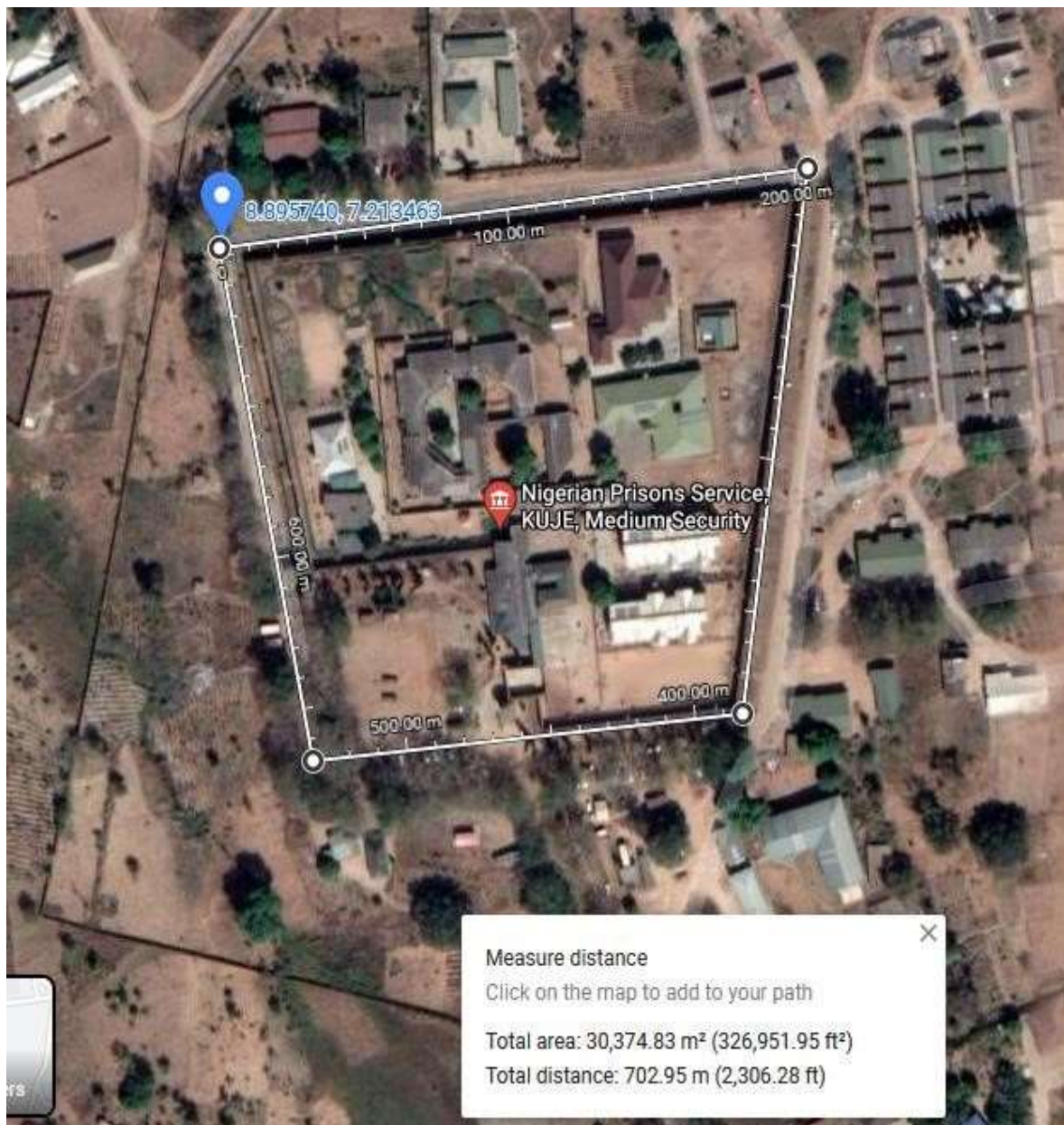
Figure 1.3: Aerial view of Kuje correctional facility
