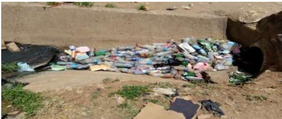
Figure 2.3: A drainage blocked with solid wastes as a result of indiscriminate waste disposal
