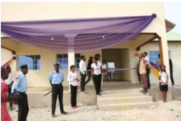
Front view of the newly constructed Search Fm Building
