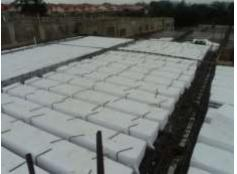
Reinforcement being fixed for an EPS slab
